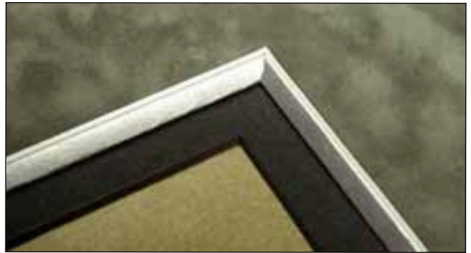
Reinforced joints are taped both vertically and diagonally with Abaca, and then burnished.
